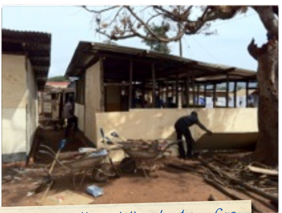
Plywood walls and tin sheet roofing.
